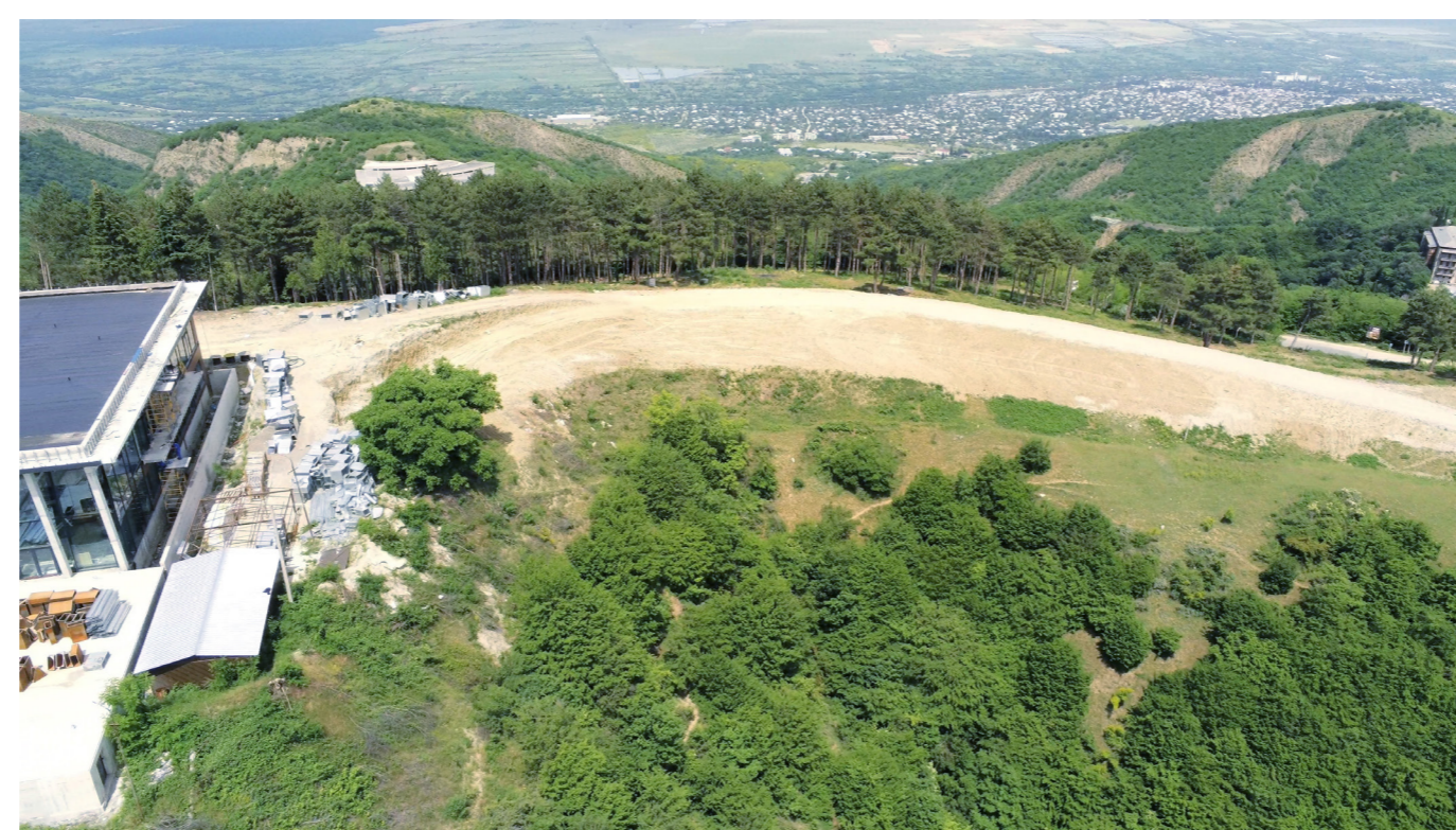
Geometrical simplicity allowed for the Sky Beach to be quickly laid out and rough graded.
